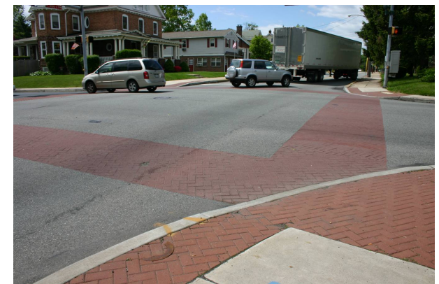
Patterned surface dressing has been applied above. It is a thin layer of aggregate that is applied directly into the roadway's asphalt surface and resembles a brick paver pattern. The painted white lines bordering the crosswalks are required on PennDOT roads. They increase visibility for vehicles approaching the intersection.
