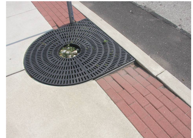
This area of the verge has sunken next to an unused tree pit. The settling of sand beneath pavers is common, so no more than a half-inch deep bed is recommended.
