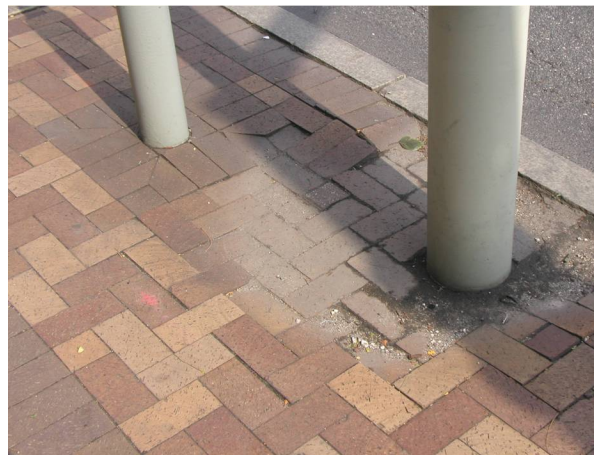
Some settling has occurred around the pole installation above. In addition to being an unsafe walking surface, the depression also allows for debris to collect.
