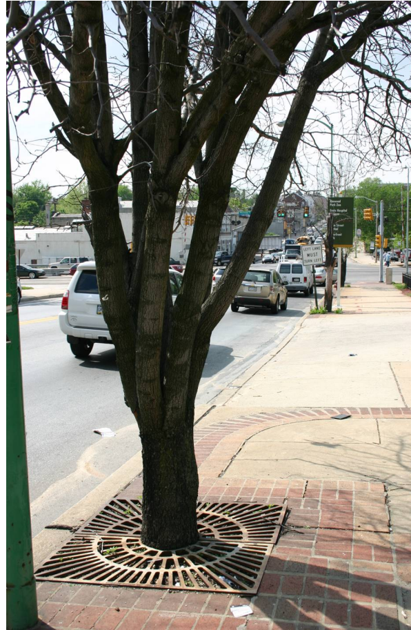
Tree grates that aren't maintained and widened over time may end up stifling tree growth. This tree grate opening is far too narrow for the size of the above tree.
