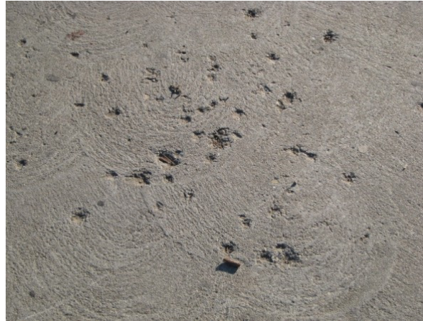
Only experienced power washers should be set loose on municipal pavement. Above is an example of what can happen to concrete when the pressure is set too high.
