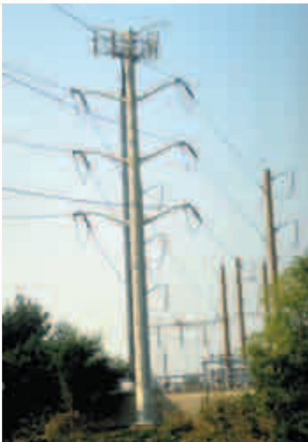
Cell tower on electric lines
