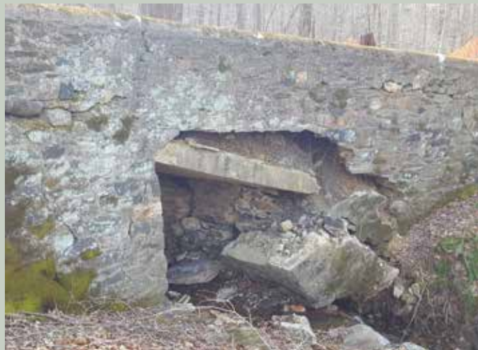
This collapsed bridge in White Clay Creek Preserve cannot be used until it is replaced. Many of the 332 bridges throughout the state park system need structural repair or replacing.
