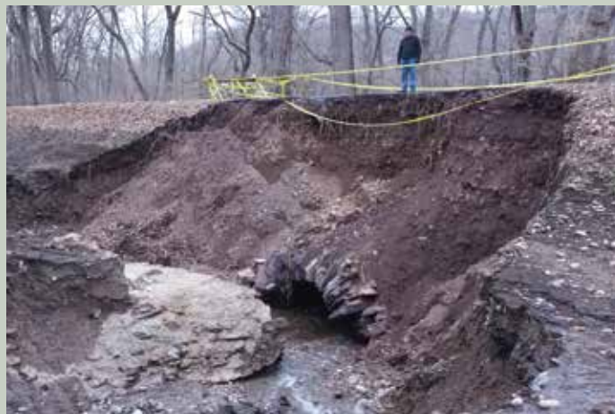
The collapse of a nearly 200-year-old culvert under the Delaware Canal in 2015 resulted in the subsequent collapse of the canal walls—an example of expensive on-going maintenance needed for historic features in many parks.
