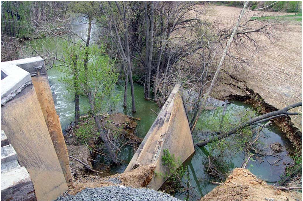
Norfolk Southern Railroad Bridge wingwall sinking into a water-filled sinkhole along Bushkill Creek
