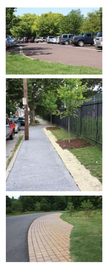
through the paving material itself or through the joints between pavers instead of running across the surface. Runoff then enters an underground stone-filled storage bed where it can be released slowly, helping to manage stormwater in a sustainable manner at its source.
