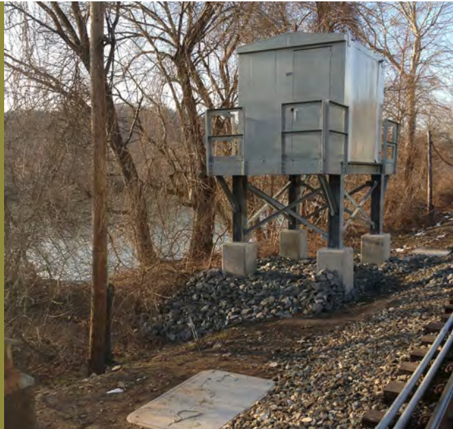
This elevated train signal hut illustrates changes designed to make infrastructure more resilient to flooding and climate change.
