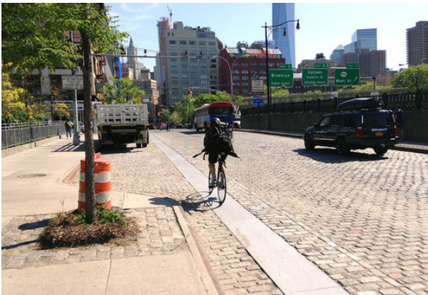
New York City Department of Transportation installed a narrow granite bike lane along a cobblestone section of Varick Street to improve comfort and reduce sidewalk riding. Photo: Brendan Klayko
