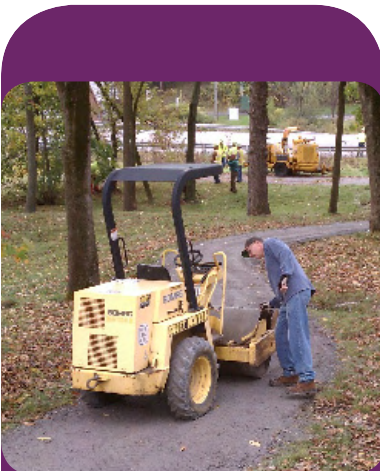
Compacting an Aggregate Tread
