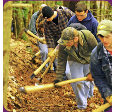
Tread Construction by Hand
