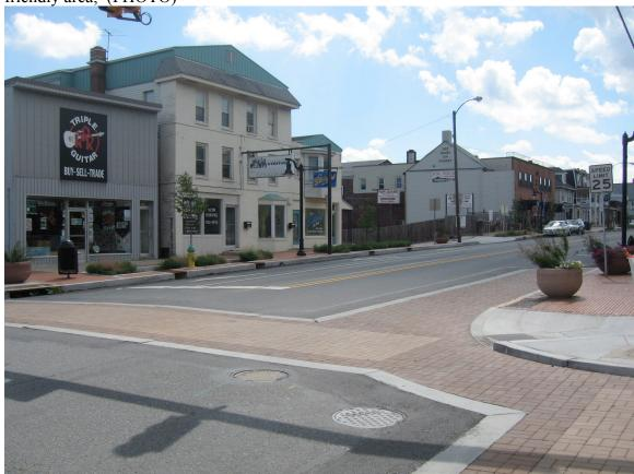
• bump outs, or curb-extensions that extend into the parking lanes but do not impact the travel lanes thus providing vertical protection for parked cars, improving pedestrian visibility and minimizing exposed crossing distances for pedestrians; and (PHOTO)
