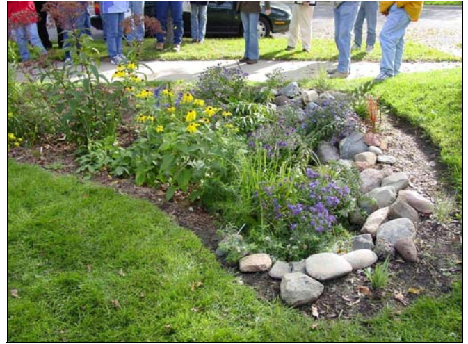
A rain garden helps stormwater infiltrate into the ground
