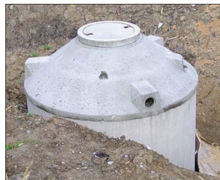
A cistern stores water underground
