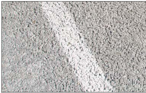
Porous concrete paving at Villanova University
