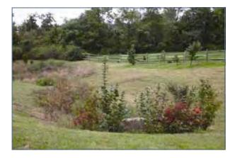
A planted stormwater basin, seen above, provides both necessary stormwater controls and an attractive amenity to the site.
