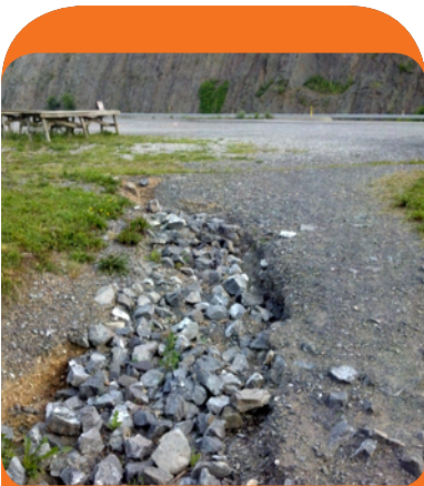
Erosion from High Velocity of Concentrated Flow
