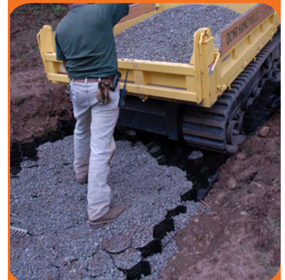
Geogrid Being Backfilled with Stone
